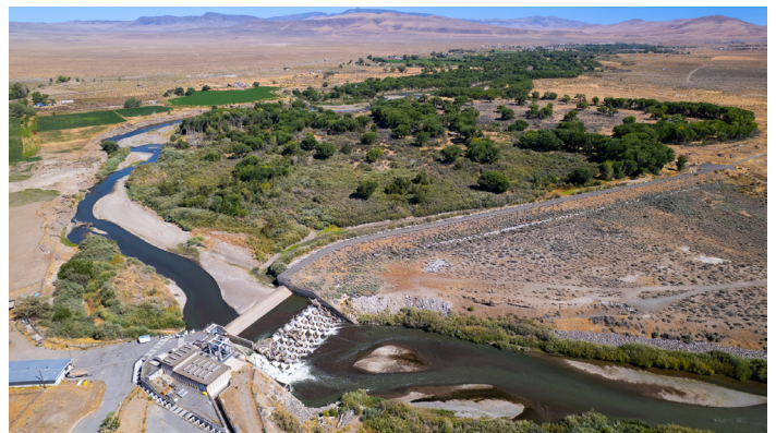
Marble Bluff Fishway provides a passage for endangered cui-ui and threatened Lahontan cutthroat trout to migrate from Pyramid Lake into the Truckee River for spawning.
